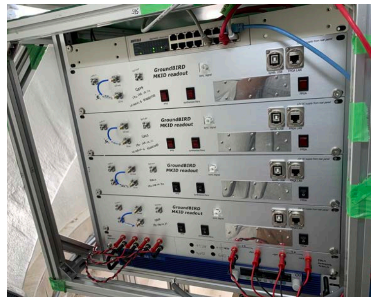
Four readout box installed!
