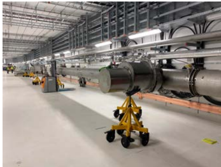
cryogenic bypass lines SIS100 placed in SIS100 tunnel, Apr'24
