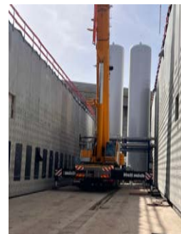
6 He tanks of the cryo facility were installed, Apr'24
