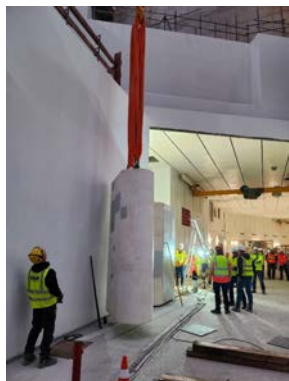
installation S-FRS lateral shielding blocks, May'24
