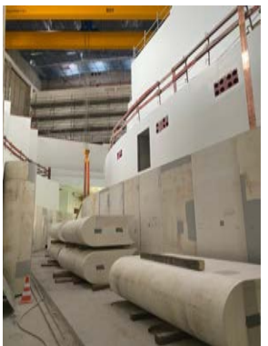
installation S-FRS lateral shielding blocks, May'24
