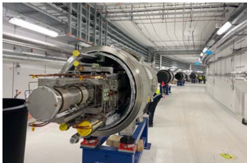
installation of SIS100 dipoles Apr'24
